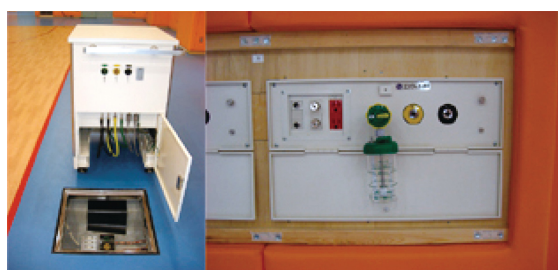
Fig. 3 Pipe Connections Embedded in Walls and Floor
